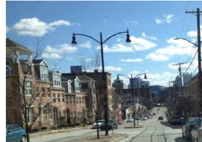
Existing lighting on Federal
