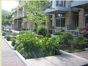
Curbside stormwater retention
